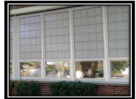
Instead of providing a separate fiberglass reinforced panel system, we can glaze a multiwall polycarbonate material within the same AW rated window system.
