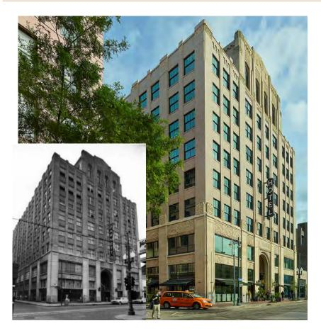
Winco's Steel Replica windows manufactured with heavy aluminum frames, making them a competitive alternative to real steel windows at a 30-40 percent cost reduction. Steel Replica windows are factory glazed and come with manufacturer's warranty. The laminated interlayer buffers noise, wind and water infiltration while offering an energy-saving 0.33 BTU/F-Hr-Ft2 U-Value. Winco offers unequal leg perimeter frames or taller profile frames for use as Steel Hung Replica windows.
