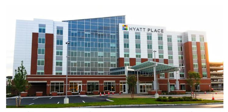
Designed for structural and thermal performance, as well as durability, WINCO's 8325 Infinity Series is an economical 3-1/4" deep strut window system. For this project, the whole window assembly needed to meet a Sound Transmission Class (STC) rating of 46. This was accomplished without the use of triple glazing or interior sashes, both of which are techniques commonly used in order to reach higher level STC ratings.
