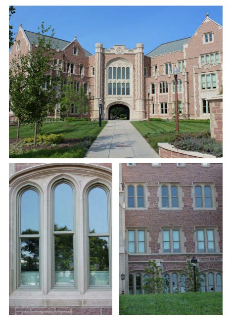
The 1450S windows are surrounded by a custom panning designed by WINCO, one of the manufacturer's specialties. A unique pre and post-set panning sets off the window's depth and integrates with the cast stonework on the façade.
